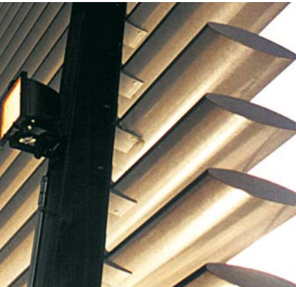
Birdsmouth brackets. Horizontally mounted csairfoil AF270 blades are shown from behind the facade of a building. Birdsmouth brackets had been fixed onto vertical support segments at specified distances and csairfoil blades were then simply slotted into the brackets and fixed with screws or rivets. Birdsmouth brackets allow for speedy onsite installations and have the additional advantage of being virtually invisible when seen from the front.
